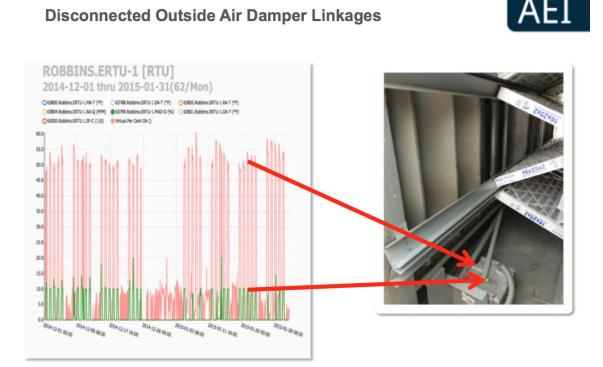
Fixing this outside air damper linkage was not difficult and resulted in both heating and cooling savings for this facility.
